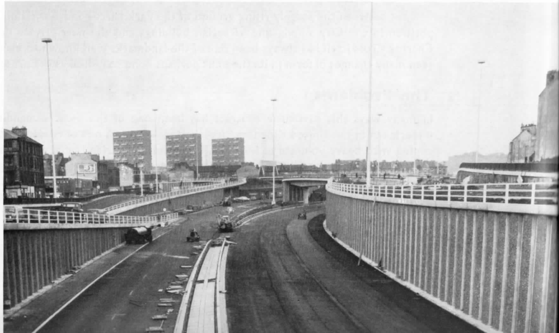
Looking North to St. George's Cross Interchange
