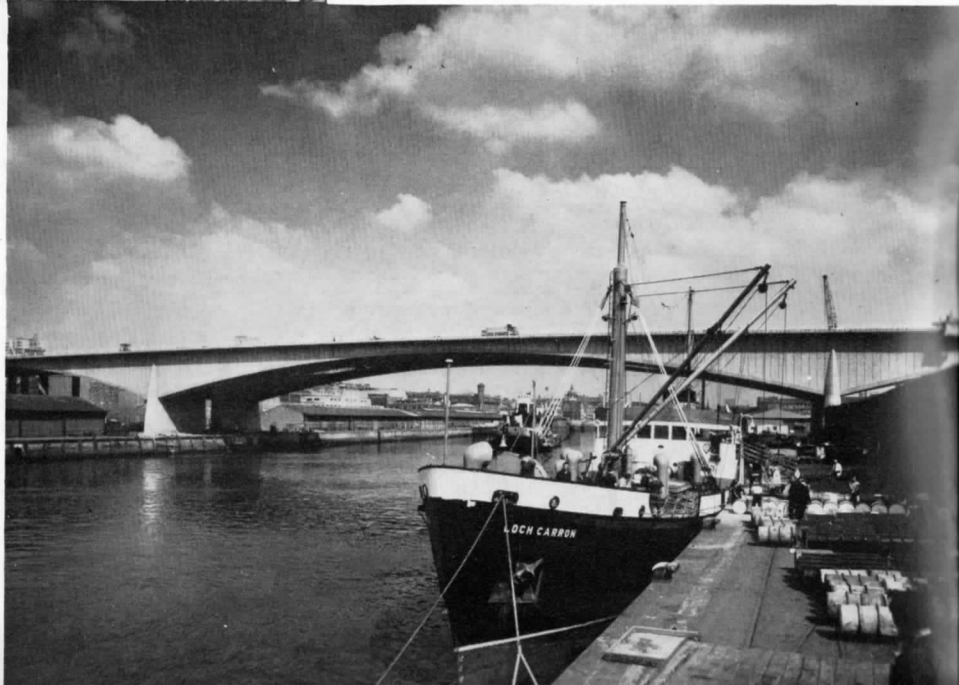
Kingston Bridge Looking Upstream
