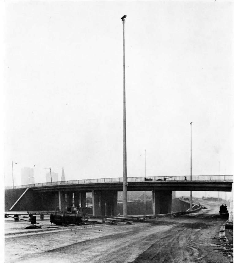
Baird Street Bridge and high mast lighting
