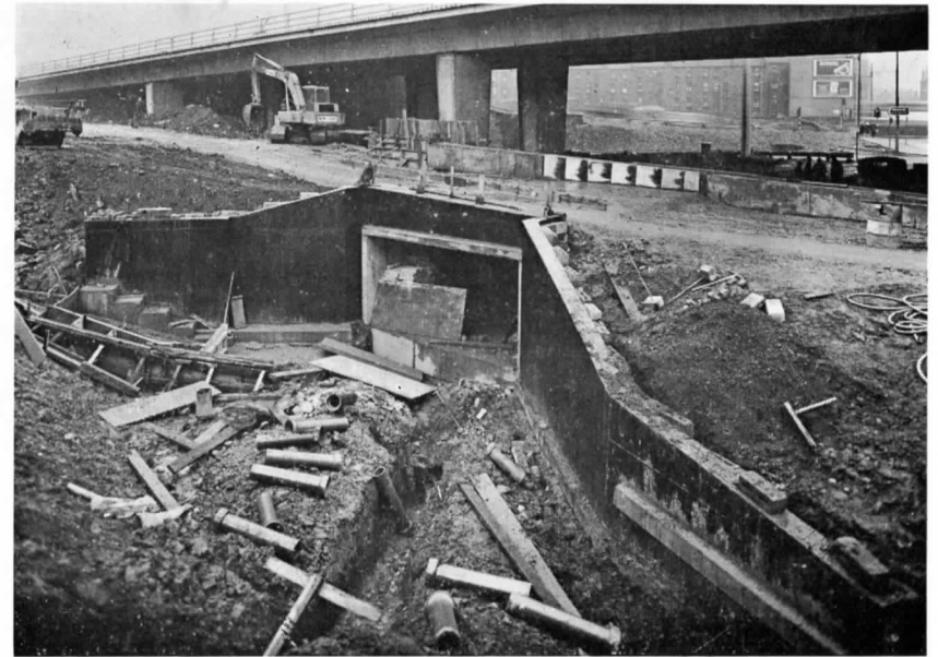
Ramps J and K East—Under construction
