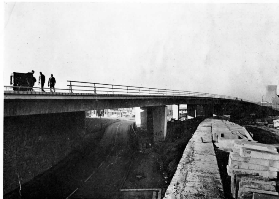
Ramps J and K East
