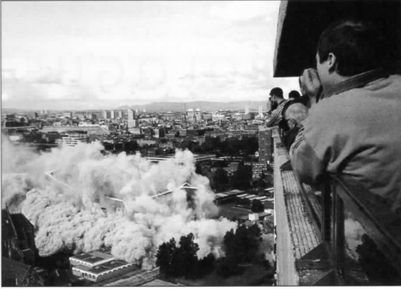
1.2 'Blowdown' of Hutchesontown 'C' on 12 September 1993.
