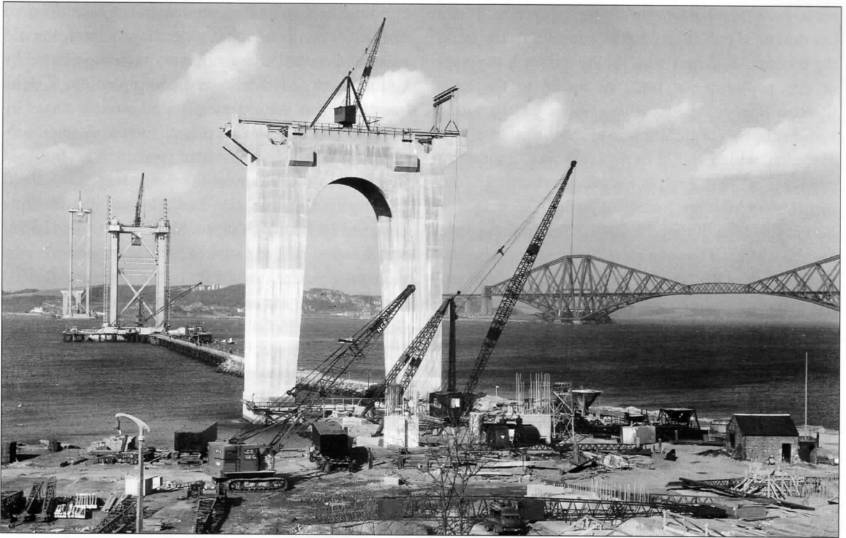
1.46 Forth Road Bridge: northward view in March 1961.
