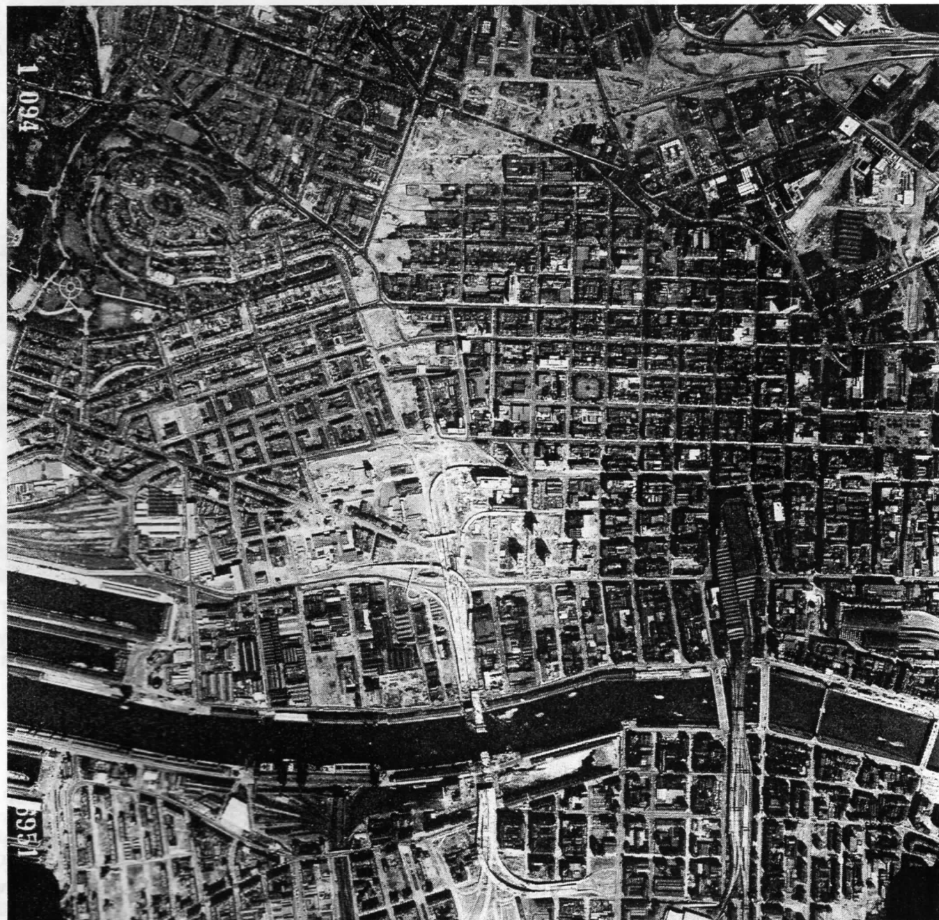
Figure 2: The Glasgow Inner Ring Motorway. Aerial view 1969 showing Kingston Bridge under construction and north flank cleared.
