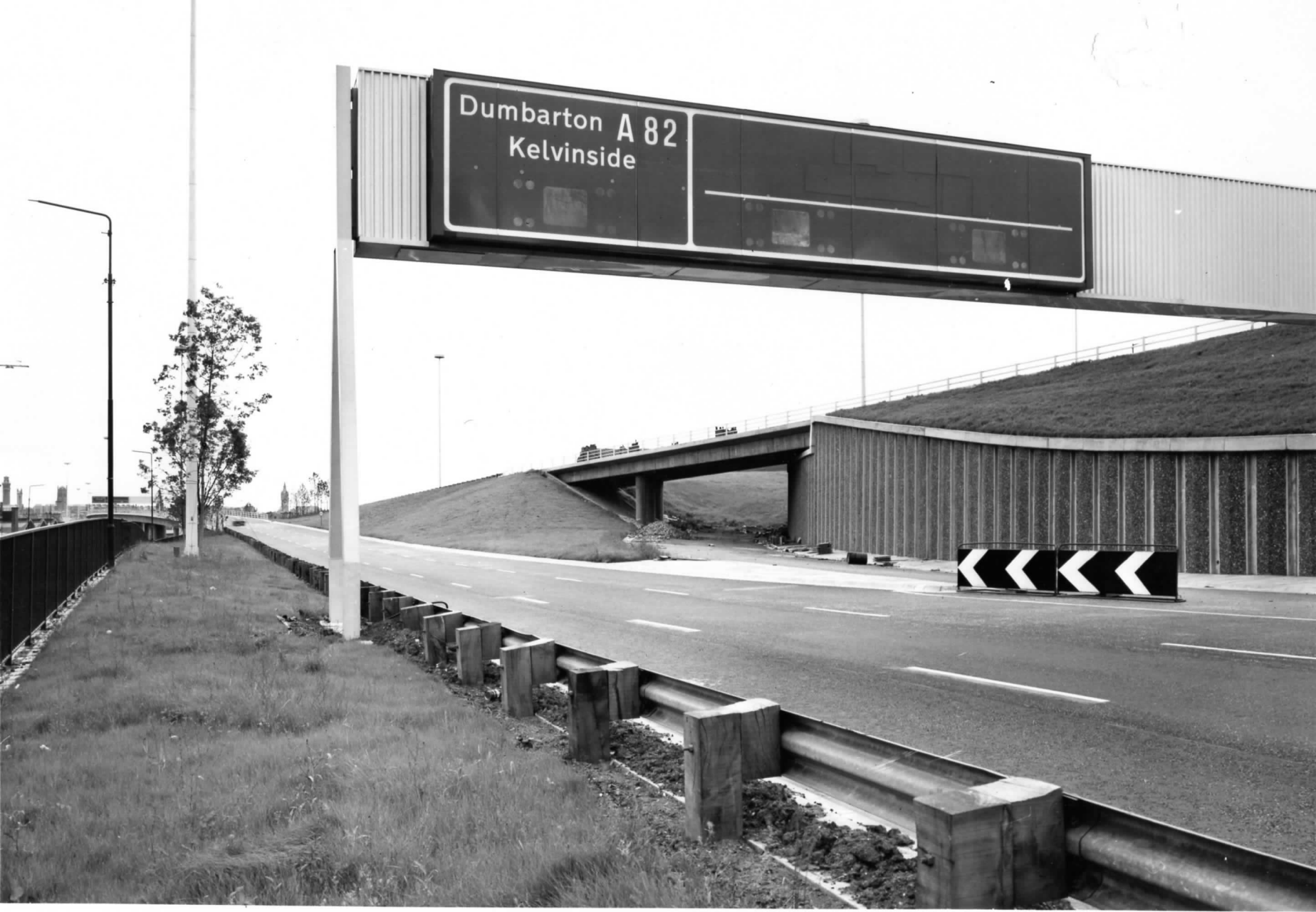
CORPORATION OF GLASGOW - WOODSIDE CONTRACT 2 Bridge 9 and Sign Gantry No. 6.
