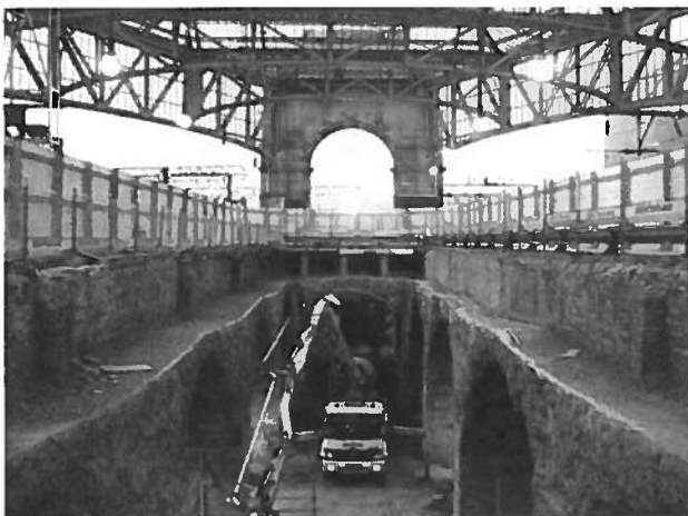
Figure 10. Excavation of the existing access ramp
