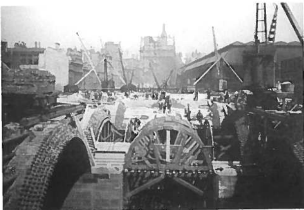
Figure 2. Construction of the arch support structures c. 1878
