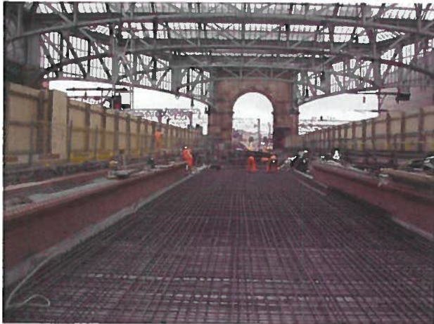
Figure 11. Construction of slab-track
