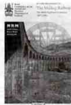
RCAHMS Mallaig Railway Broadsheet – Glenfinnan Viaduct with the timber centering used to build it © RCAHMS [ISBN 1902419316]*
