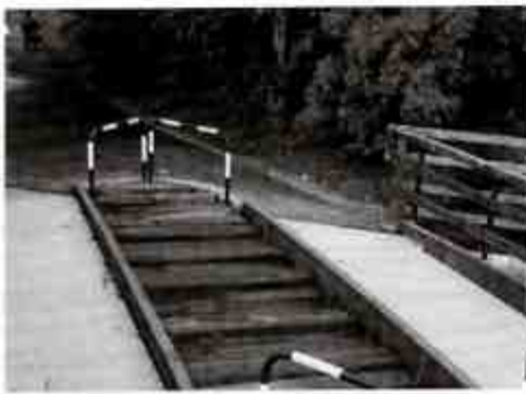
Braid Burn Bridge after being raised 0.9m – September 2001 © The City of Edinburgh Council
