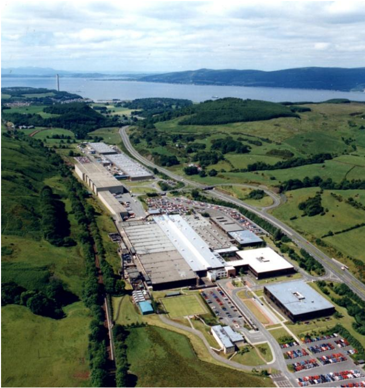
IBM Greenock looking west down Spango Valley towards the Inverkip Chimney
