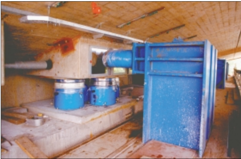
Fig 5. Hydraulic jacking systems B and C
