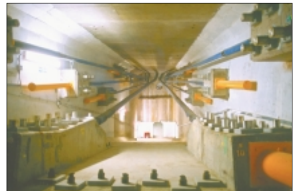
Fig. 4. External prestressing tendons retrofitted inside the existing bridge deck voids
