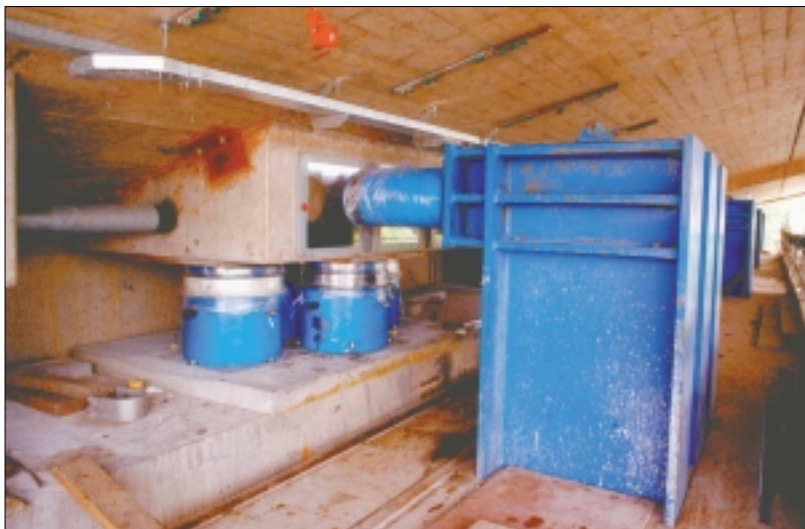
Fig 5. Hydraulic jacking systems B and C
