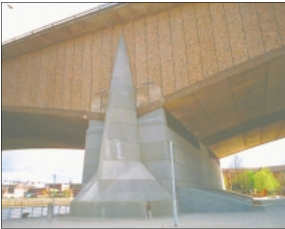
Fig 8. After installing the new bridge bearings
