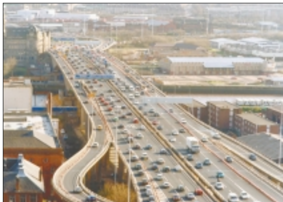
Fig. 3. Lane restrictions and concrete blocks during the works
