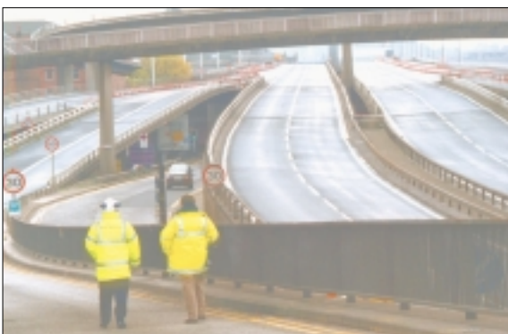
Fig 6. The motorway was totally closed during jacking operations
