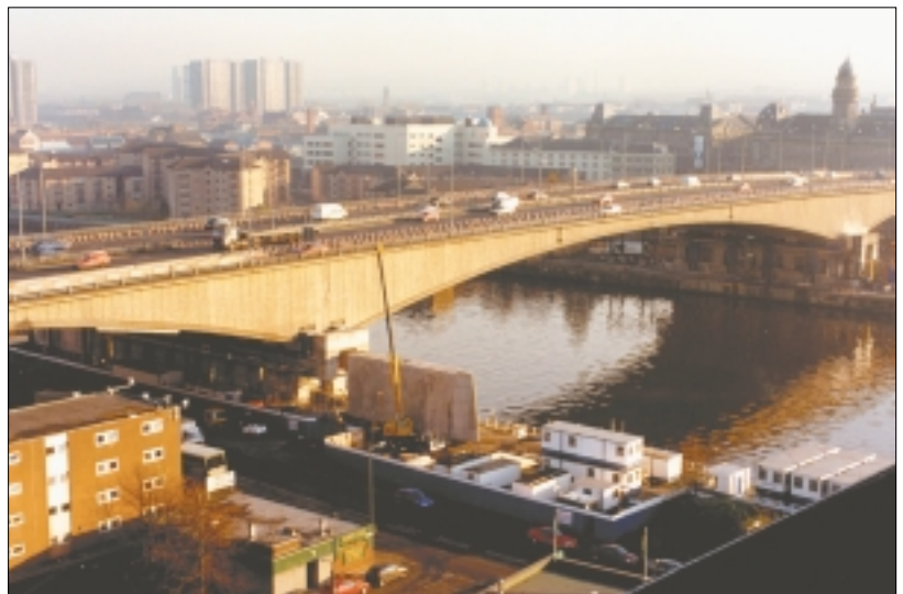
Fig 7. Existing pier slid out from below bridge
