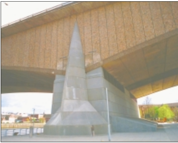
Fig 8. After installing the new bridge bearings
