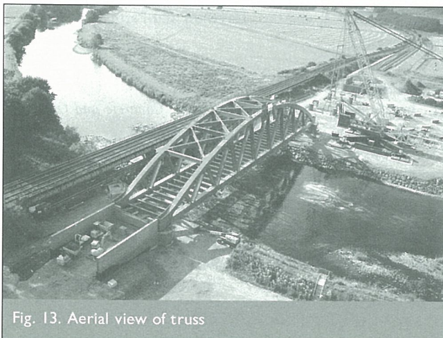
Fig. 12. Truss girder erected over the River Nith
