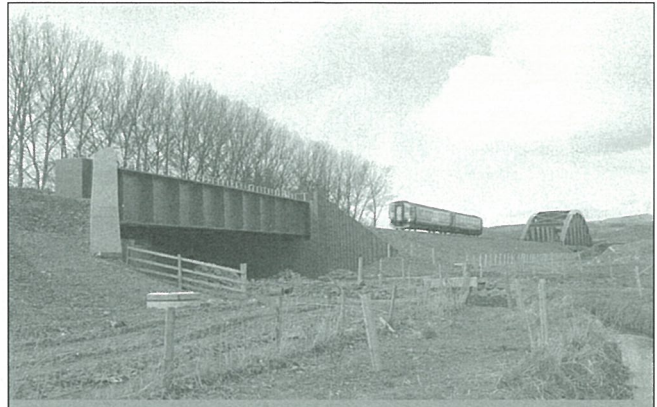
Fig. 18. The completed realignment
