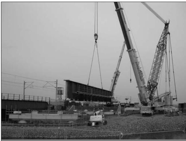
Fig. 8. February 2006—the first main girder section is lifted in
