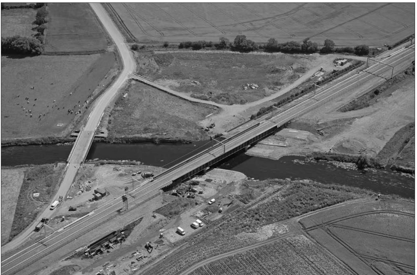
Fig. 12. Aerial view from the north bank. The diverted stream is visible on the right
