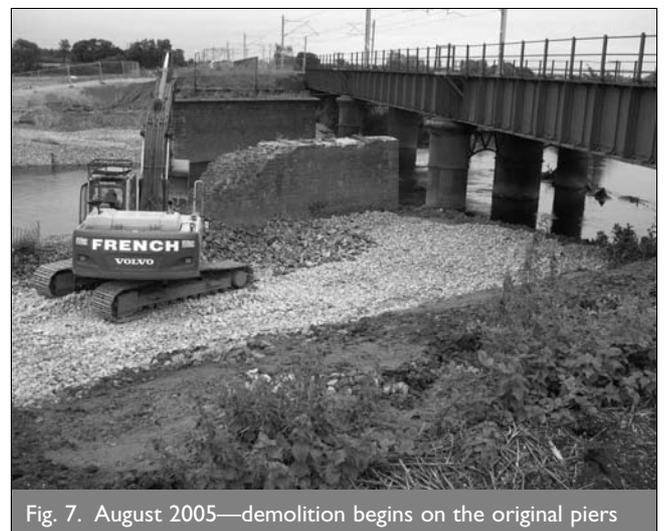
Fig. 7. August 2005—demolition begins on the original piers
