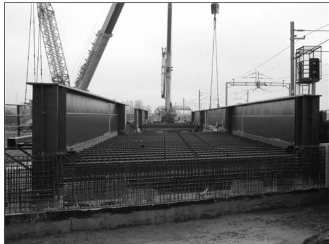
Fig. 9. Cross-girders and shear studs
