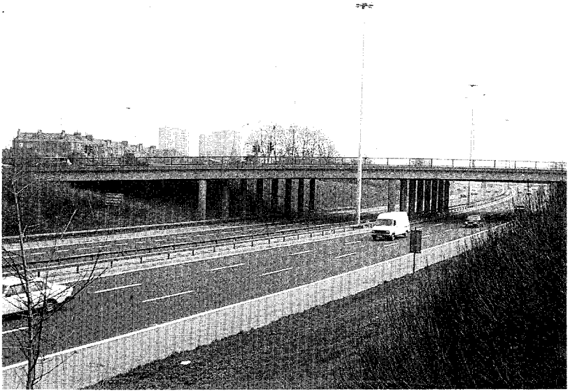
Renfrew Motorway — Stage 1: Dumbreck Road Bridge
