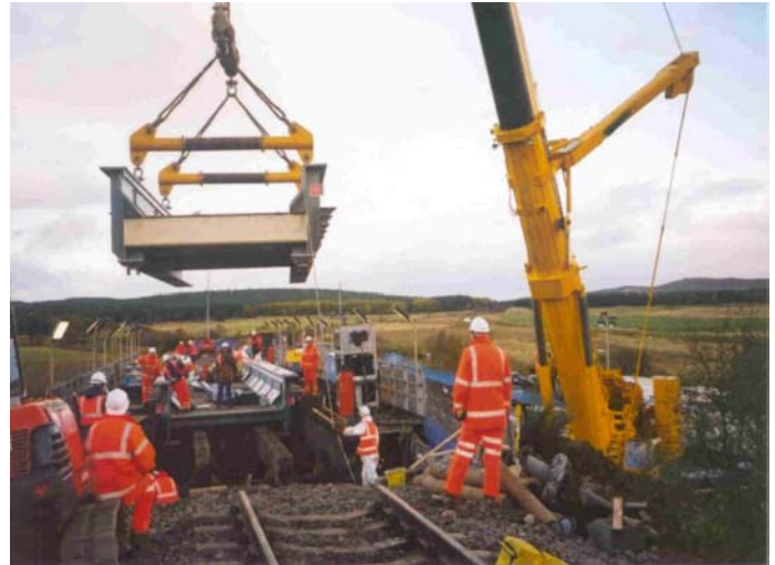
Installation of Moy Viaduct Superstructure
