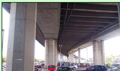
We are working on two aspects of **White Cart Viaduct** on the M8 at Glasgow Airport – the design and contract documentation for the installation of high-containment parapets and replacement lighting columns, and more recently a major new commission – the design of a strengthening scheme for the steel box girders and deck cantilevers. This follows on from similar strengthening and repair work on the **M74 Raith Bridge**.
