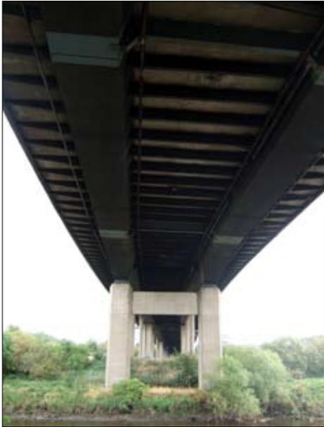
We have been involved in work on the M8 White Cart Viaduct at Glasgow Airport since undertaking a structural assessment in 1997. Originally constructed in 1968, the 23-span steel/concrete composite box girder viaduct carries around 80,000 vehicles per day and is now undergoing a phased programme of strengthening and refurbishment.
