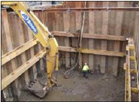
photograph, taken on 13th June 2008, shows preparations being made for the third and final level of frames. Excavations were hampered by twin fibre-optic cables, heavy ingress of water and the 1870's equivalent of Irn Bru cans. Collectors' pieces of ironstone are available. The fabrication of the super-structure, is shown in the photograph below. With the project running to
