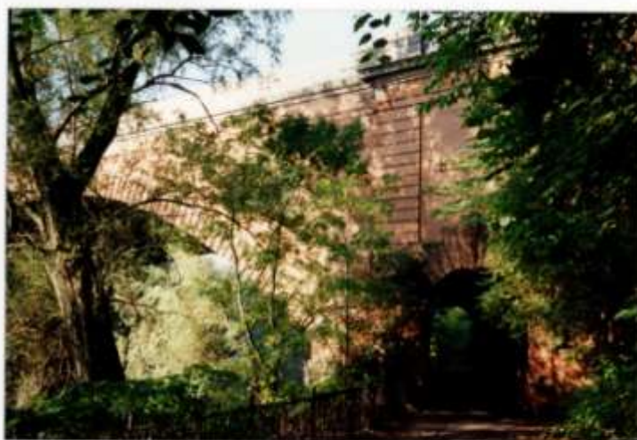
QUEEN MARGARET BRIDGE GLASGOW 1926
