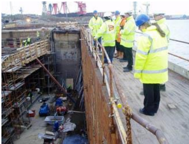
View from the dock gate of one of the concrete boxes in the dry dock
